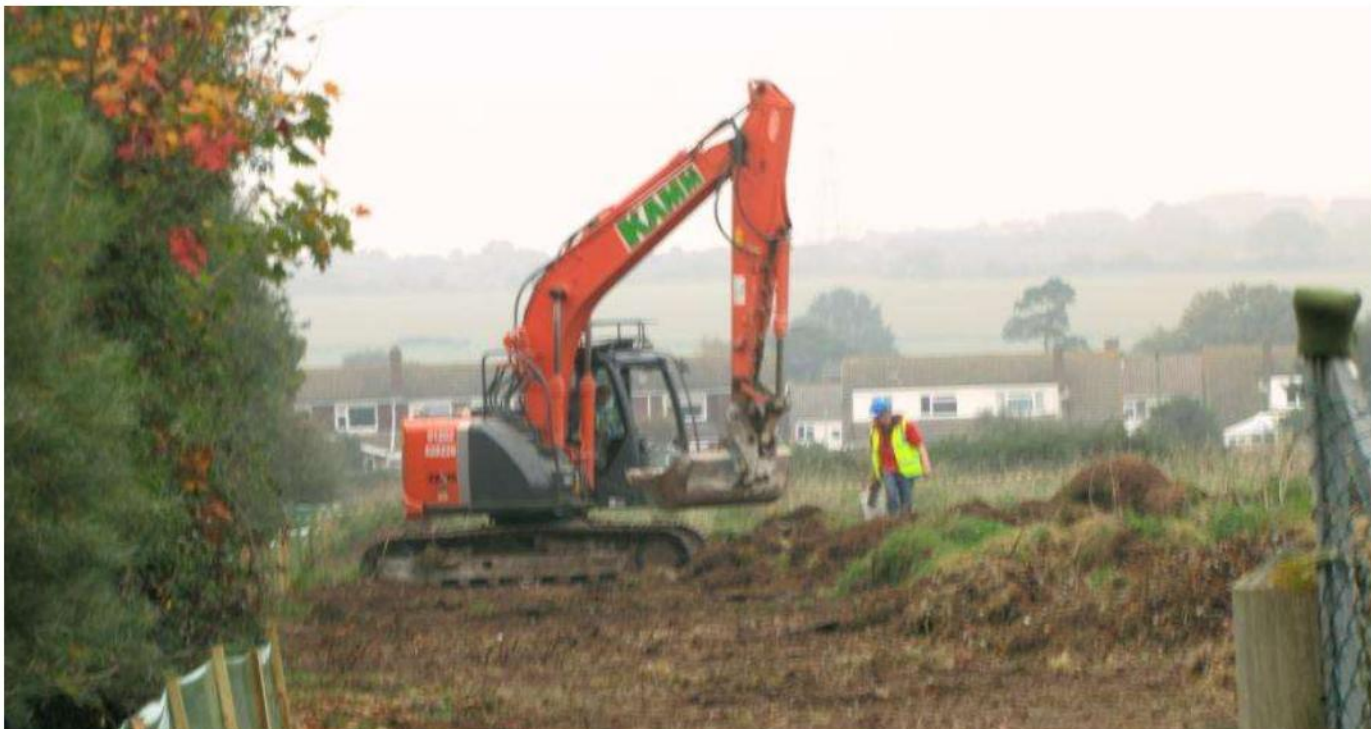
Fig. 3 Earthworks, photograph taken October 2017.
