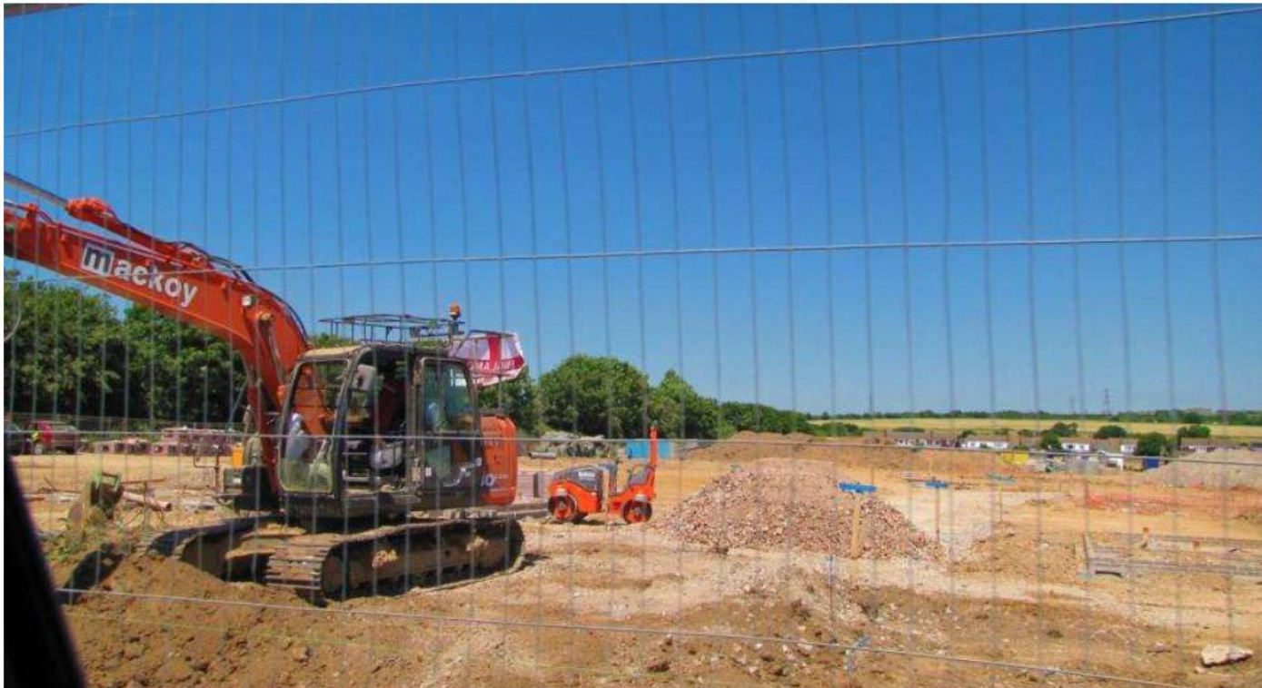
Fig. 7 Immediately below, typical works being carried out, (Area Map 7)
